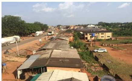
Plate 1: Construction of shops on drainage area
