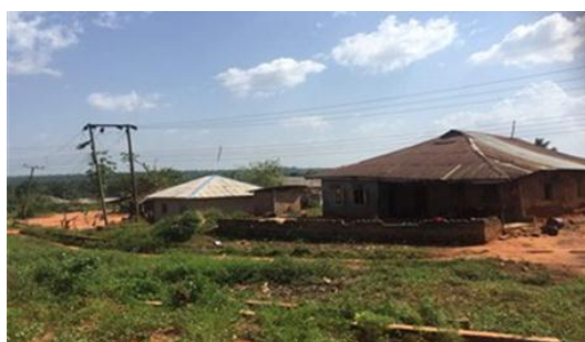
Plate 2: Condition of existing road
