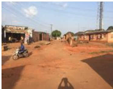
Plate 8: Existing road condition
