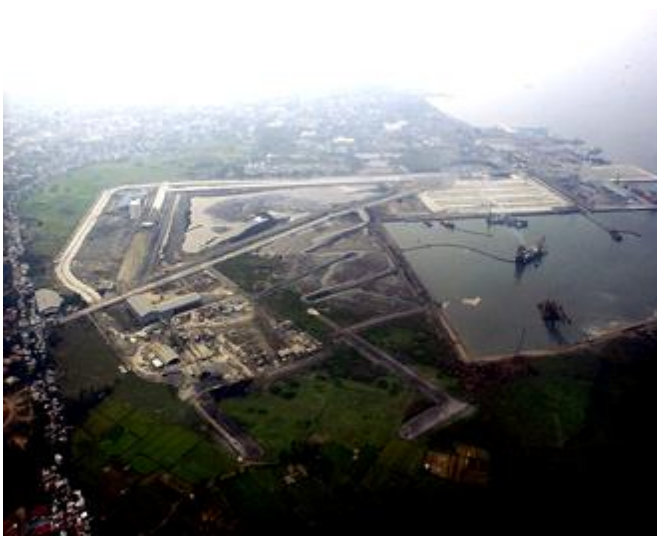
Overall View of Batangas Port Phase II covering an Area of 128 hectares with an Estimated Cost of P7 Billion
