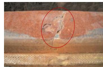
Figure 14: Rail Head Metal Spalling in the Gap between Adjoining Rail at IRJs
