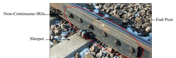
Figure 9: - Non-Continuous Supported IRJs [16]
