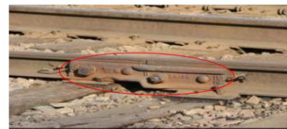
Figure 3: Compromise Joint Bar
