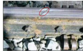
Figure12: Rail End Metal Flow Figure13: Schematic Diagram of Rail End Metal Flow. It can lead to the development of further damage such as spalling as shown in Figure 14. Key factors associated with this type of failure are rolling contact fatigue and the associated loading rate dependent metal plasticity as the wheel load exceeds the material yield point at the point of contact.
