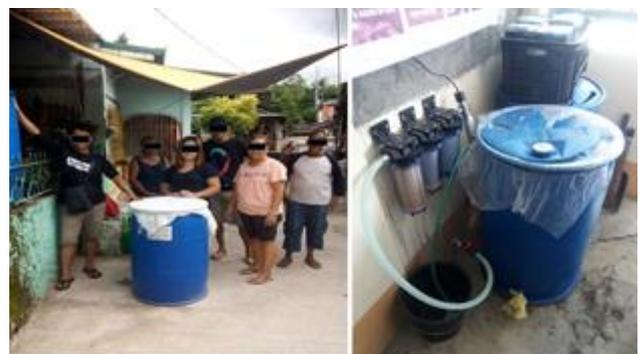
**Figure 13:** Improvised rainwater collection using tarpaulin and drum
